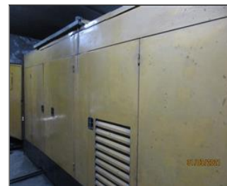
External photo(s) of the production unit(s) Generator.JPG
