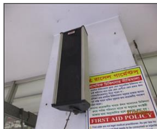
Photo of the inside of the main production hall Public addressing system.JPG
