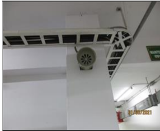
Photo of fire safety equipment Fire alarm bell 2.JPG
