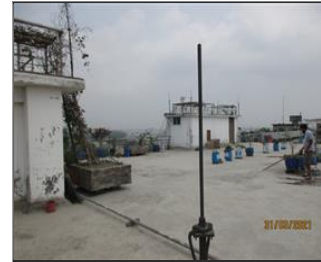
External photo(s) of the production unit(s) Lighting protection system.JPG
