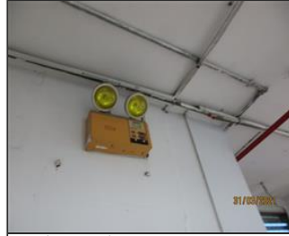
Photo of the inside of the main production hall Industrial battery backup fog light.JPG
