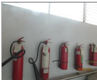
Photo of fire safety equipment Fire extinguisher.JPG
