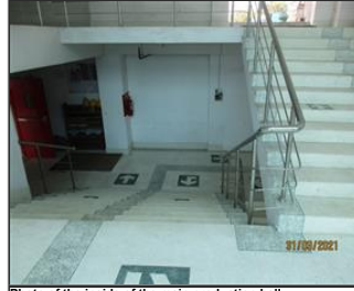
Photo of the inside of the main production hall Main staircase.JPG
