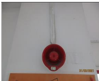
Photo of fire safety equipment Fire alarm bell 1.JPG
