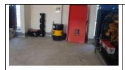
No secondary containment under diesel oil drum
