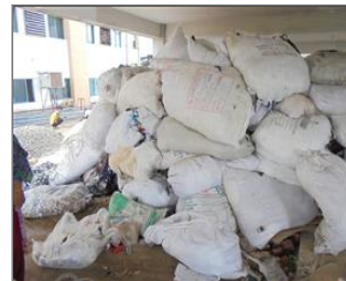
Photo of non-conformity Wastage were not segregated.JPG
